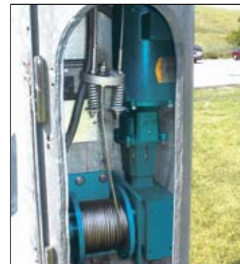
Internal Motorized Hoist (HIM Option)
