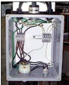
NEMA 4 junction box (Mounted to ring)
